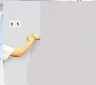
All walls and floor must be primed before tanking.
