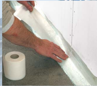
Reinforcement is fixed with LIP VS 30.
